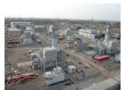
Fast Track Project for three gas turbine power plants is aimed at the installation of eight new gas turbines in the three different Iraq sites of Karbala, Hilla and Taji, for a total capacity of 660 MW.
